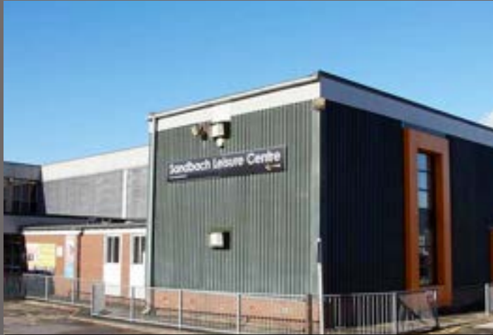
Sandbach Leisure Centre Gym, sports hall & swimming pool
