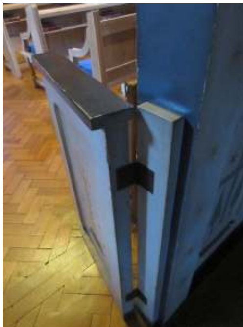
The west screen gates.
