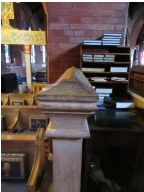
Top & end-rail of low screens in N arches.
