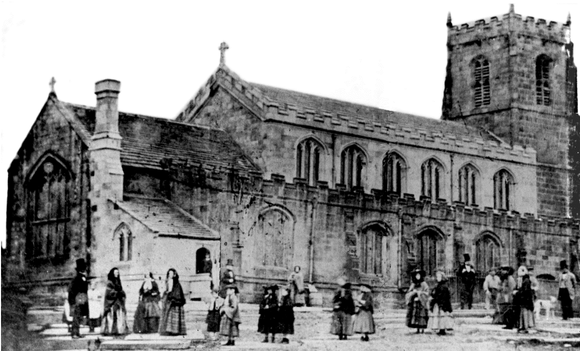
North view shortly after the 1855 restoration, clearly showing the new, lighter stonework
