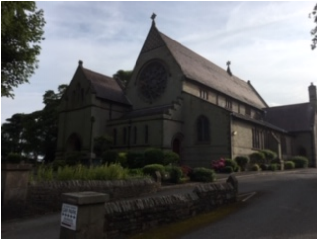
All Saints' Church general view front/west elevation
